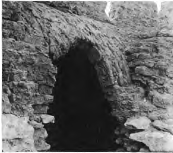
(a) View of vaulting to the south aisle from the Haikal.
